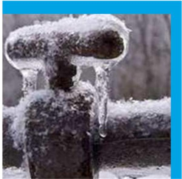
must be known by key personnel in order that the water supplies can be isolated immediately should there be a problem. These valves should be exercised on a regular basis in order to ensure that they remain operational.
