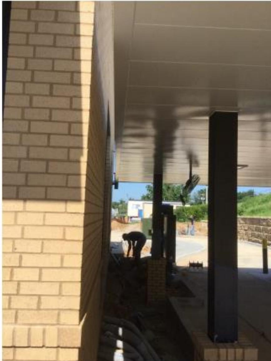
Photo 1 - Noncombustible Drive Thru Canopy (Note: Canopy Not Attached to the Building)
