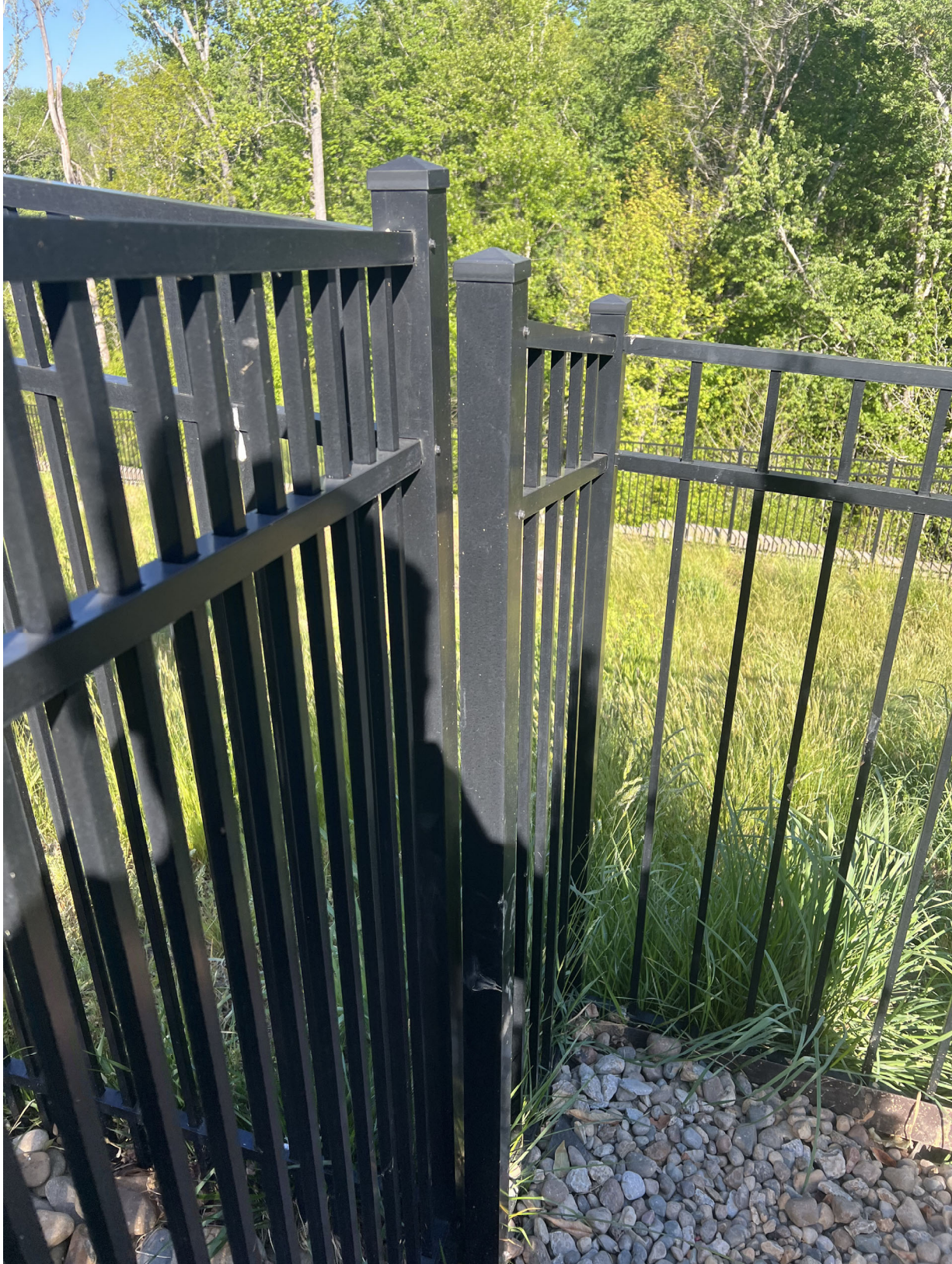
Photograph 2. Fence Rear — Submitted photograph showing the rear portion of the fence located along the adjoining property.
