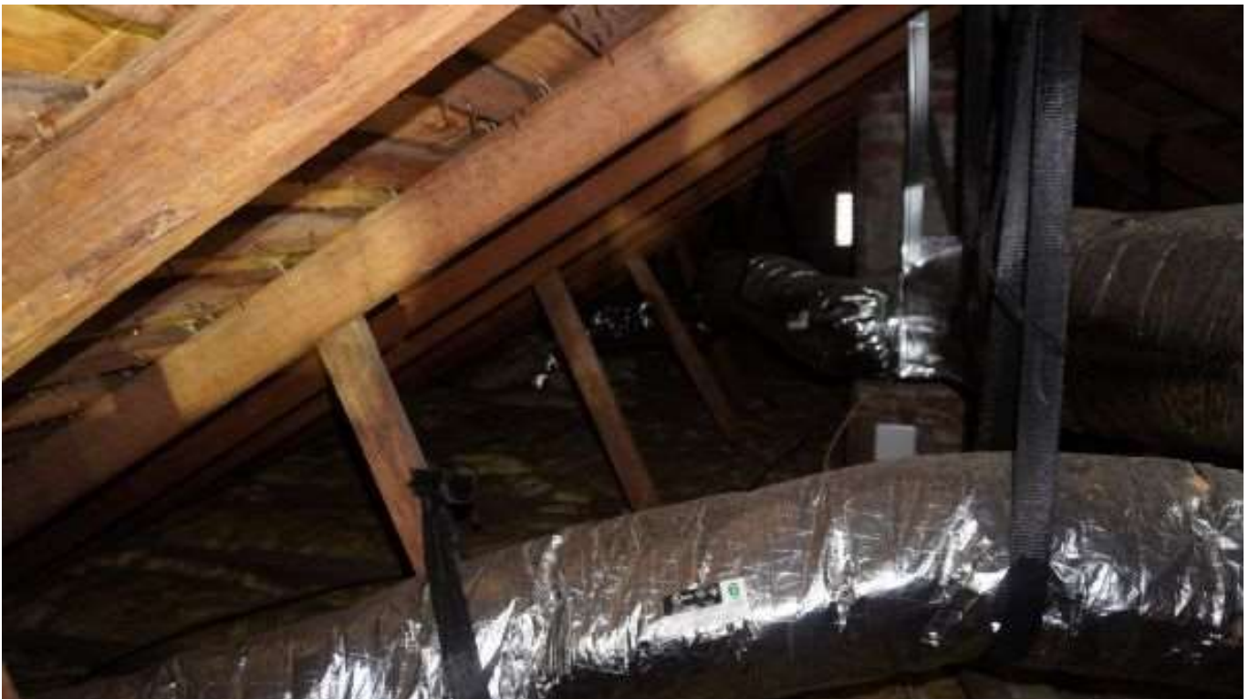
Below: Attic – roof framing with knee braces at rafters visible
