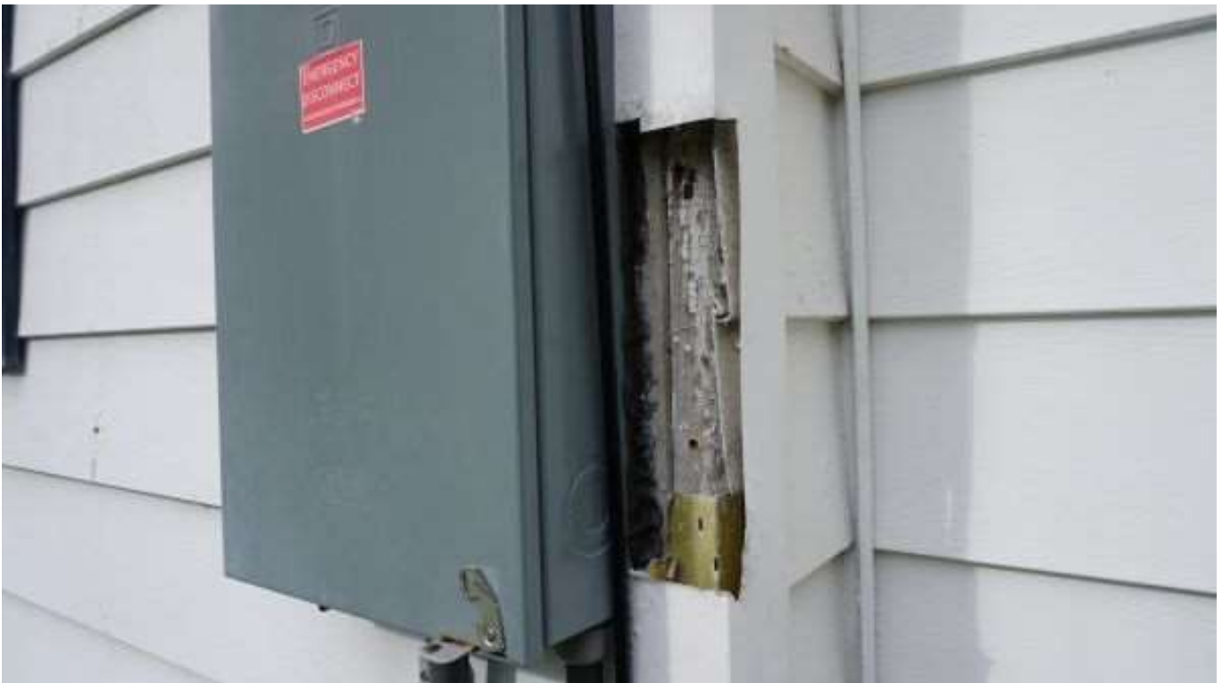
Below: Right elevation – missing trim at building corner – older cladding layers visible
