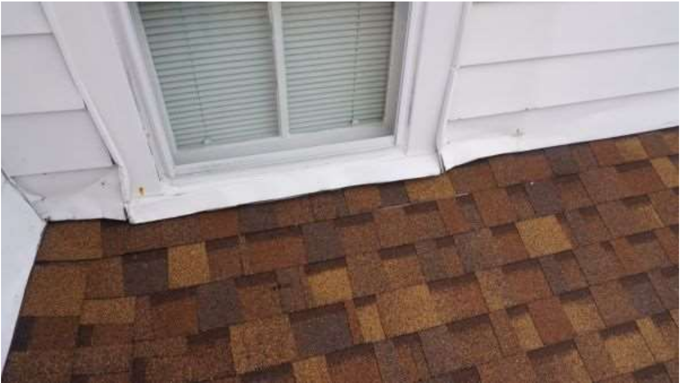
Below: Front porch roof – window trim and siding damaged by flashing replacement
