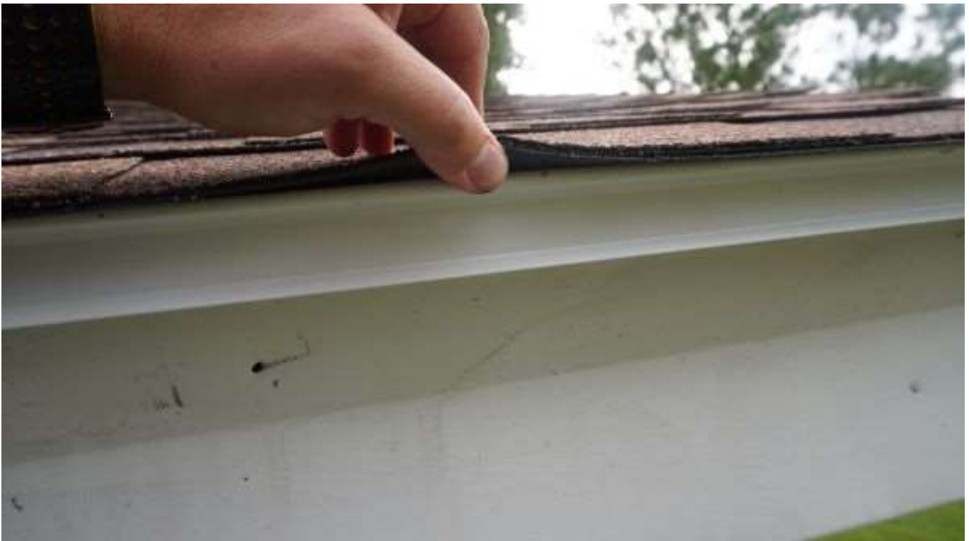
Below: Front porch roof – drip edge present
