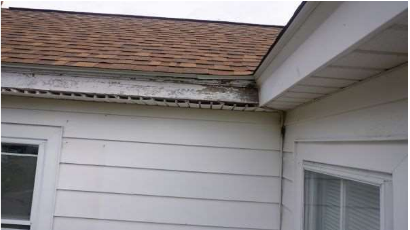
Below: Front porch roof – fascia condition where trim missing
