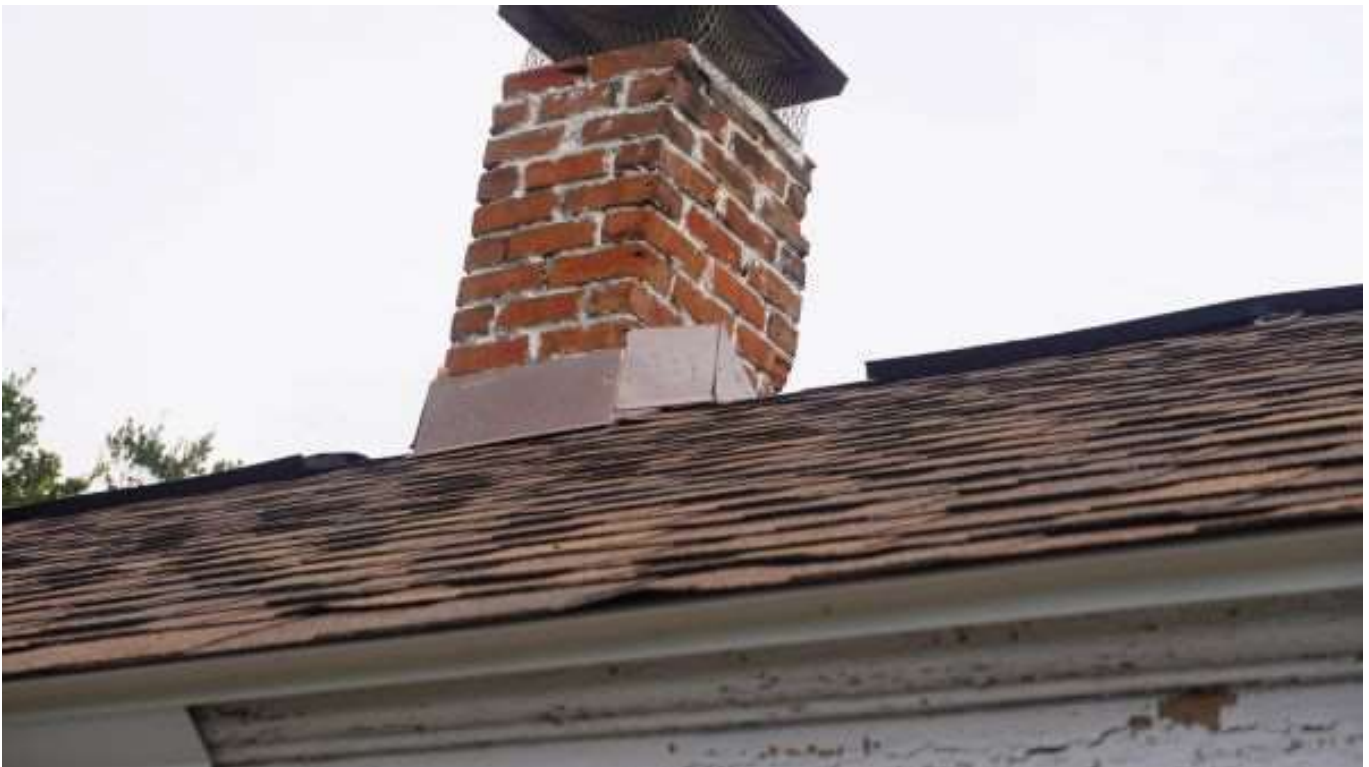
Below: Main roof – copper chimney flashing
