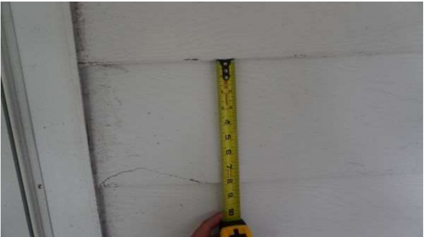
Below: Front elevation aluminum siding exposure
