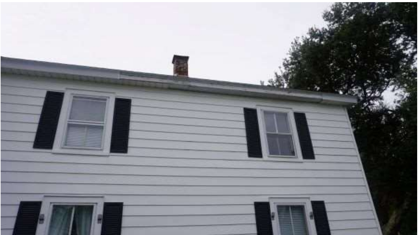
Below: Rear elevation – fascia and soffit missing
