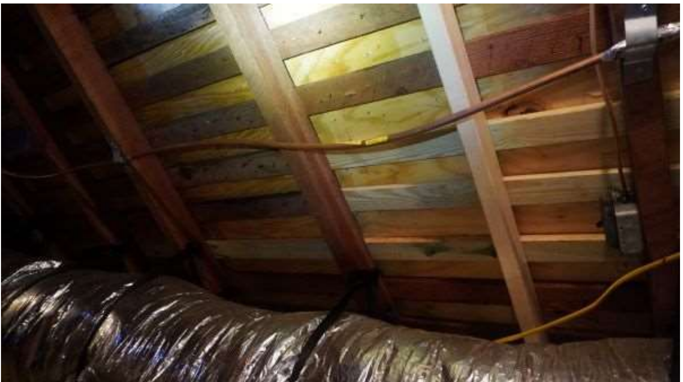
Below: Attic – Roof farming with spaced and solid decking visible
