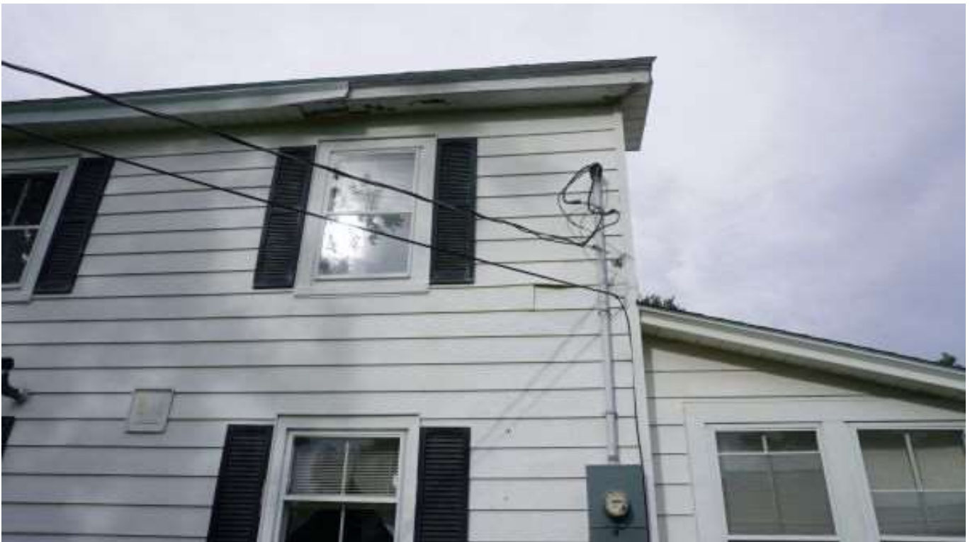
Below: Right elevation – siding, trim, and electrical mast damaged due to tree limb impact
