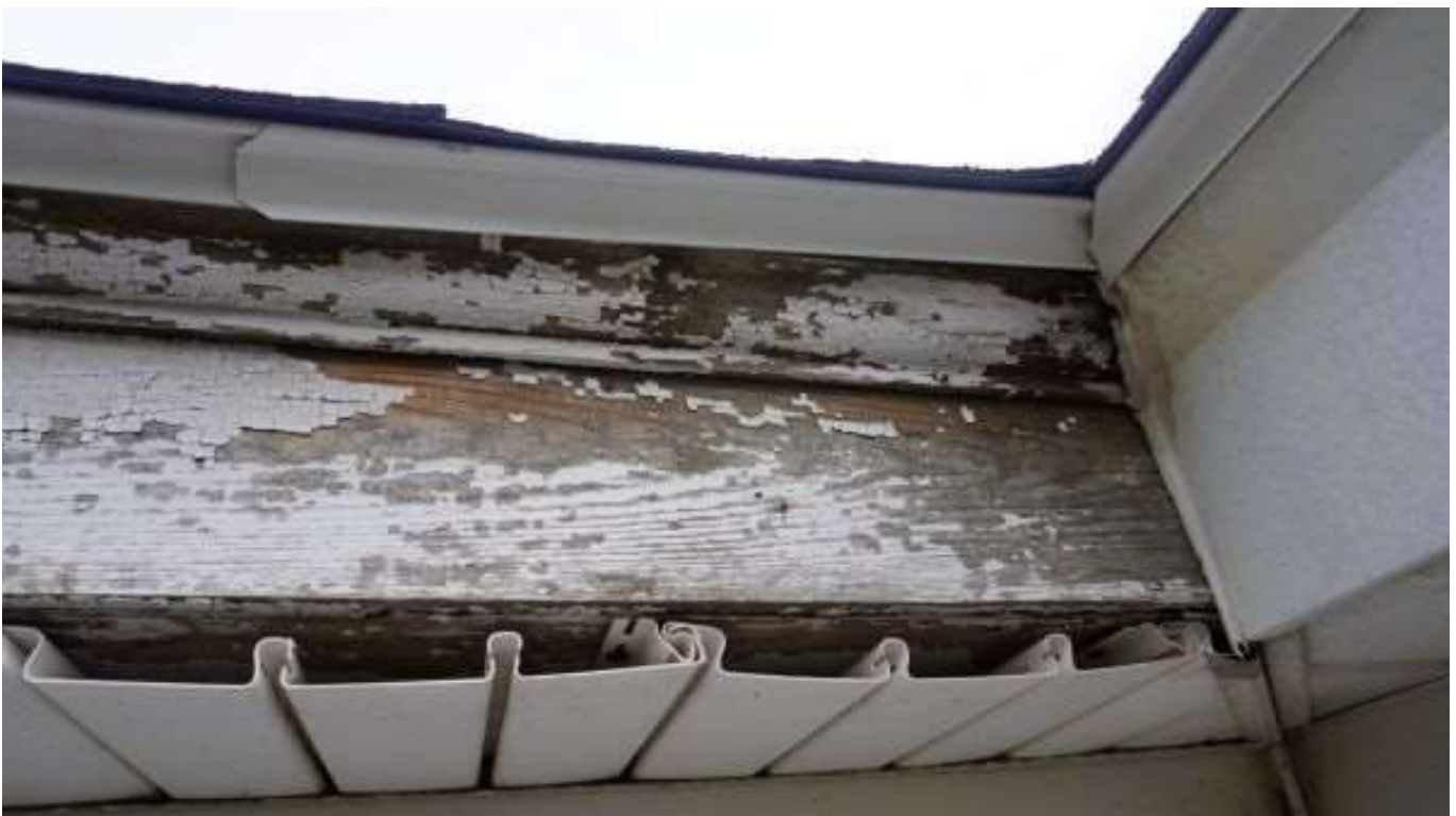
Below: Front porch roof – fascia condition where trim missing
