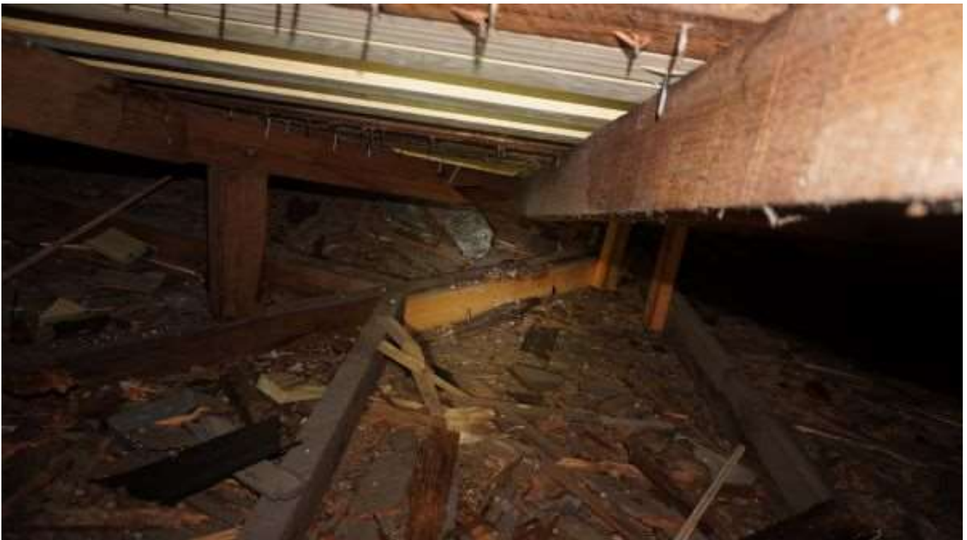
Below: Interior – upstairs hallway – paneling removed – porch roof framing visible
