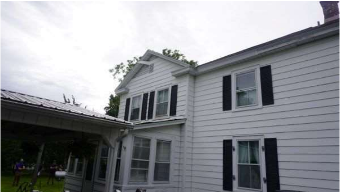
Below: Rear elevation – siding damaged at roof-wall intersection from roofing replacement
