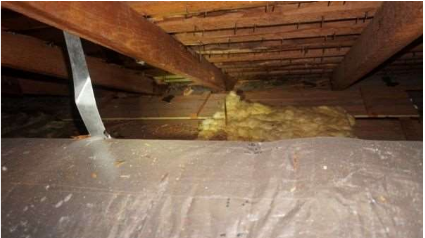
Below: Attic – roof framing with knee braces at rafters visible
