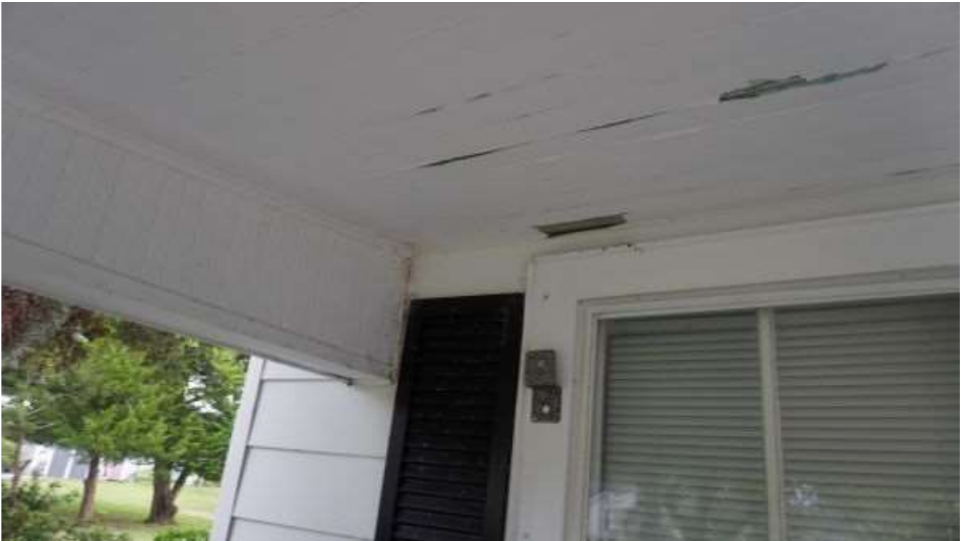
Below: Front elevation – missing fascia trim on gable
