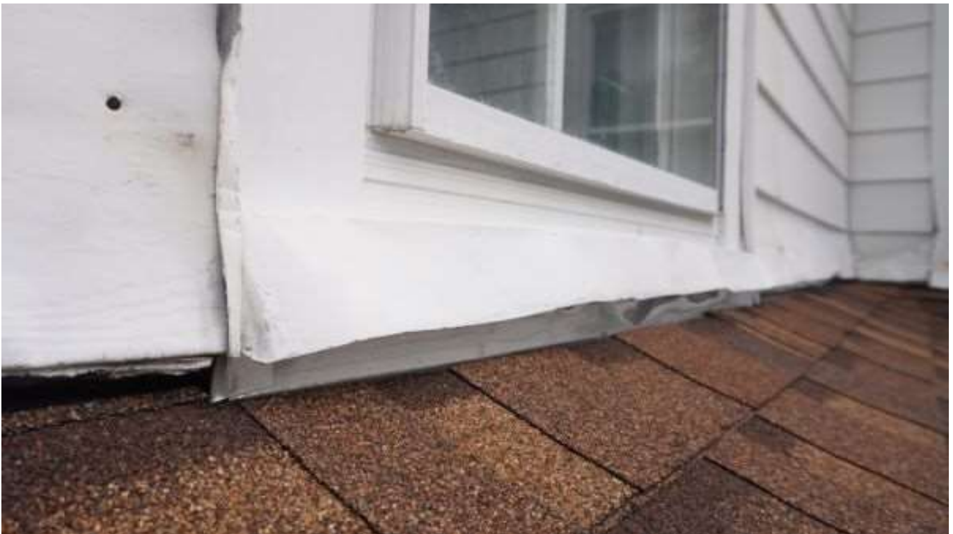
Below: Front porch roof – window trim and siding damaged by flashing replacement
