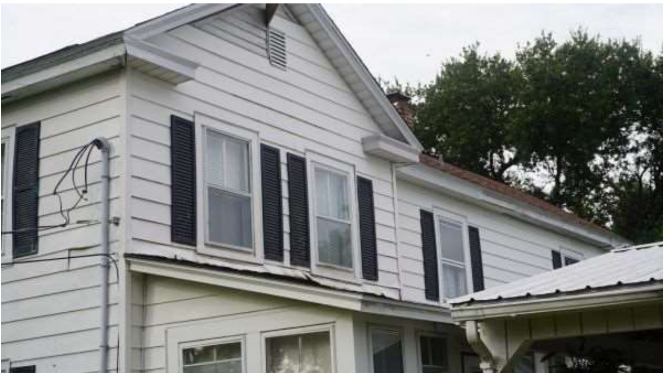
Below: Rear elevation – damaged siding at peak of gable
