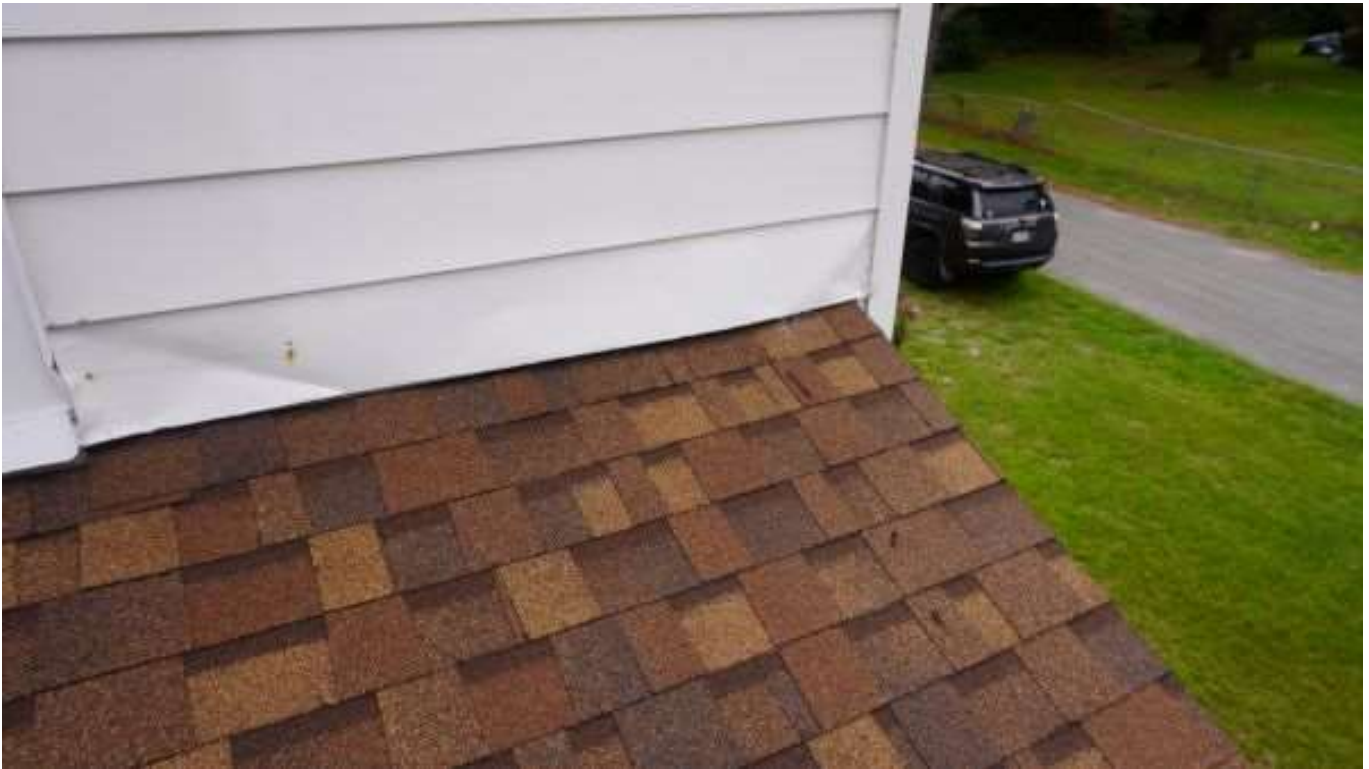
Below: Front porch roof –wall siding appears newly installed
