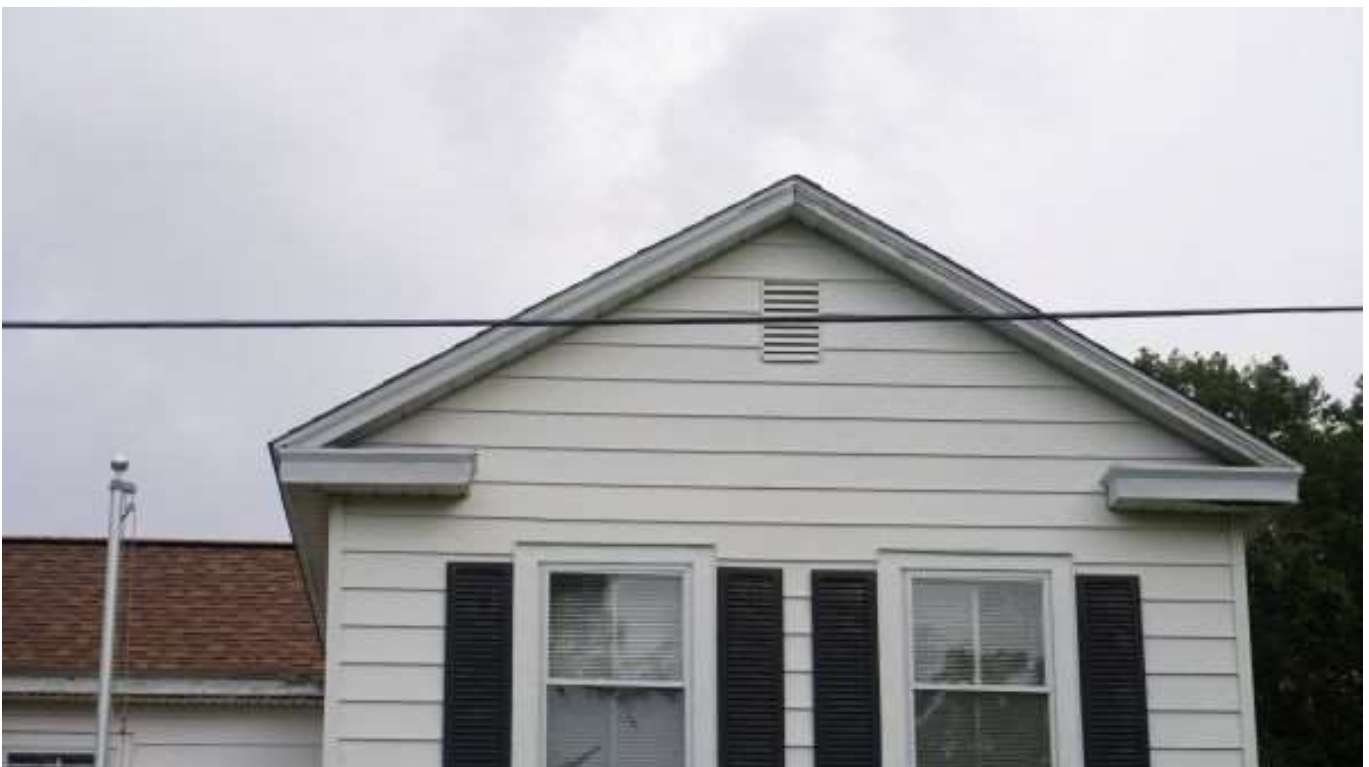
Below: Front elevation – missing fascia trim on gable
