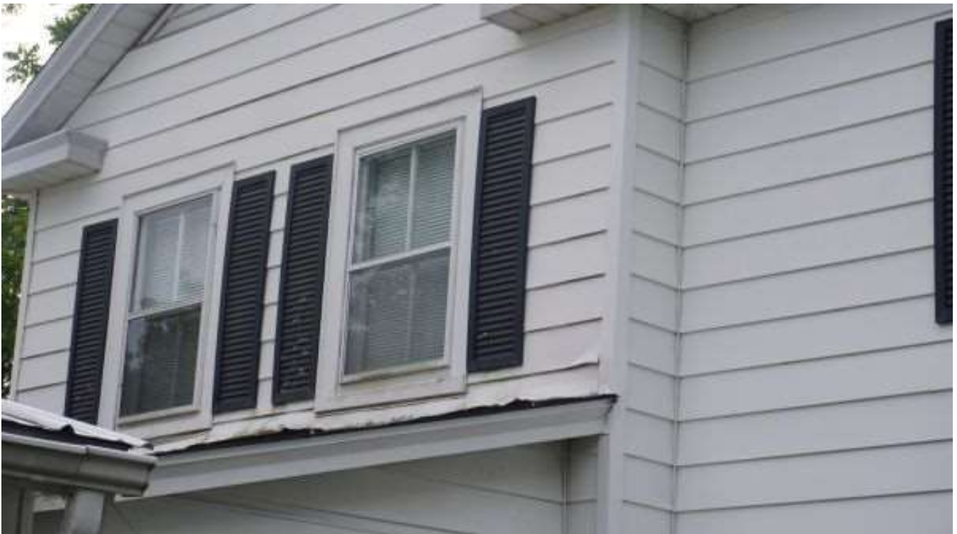
Below: Rear elevation – siding damaged at roof-wall intersection from roofing replacement
