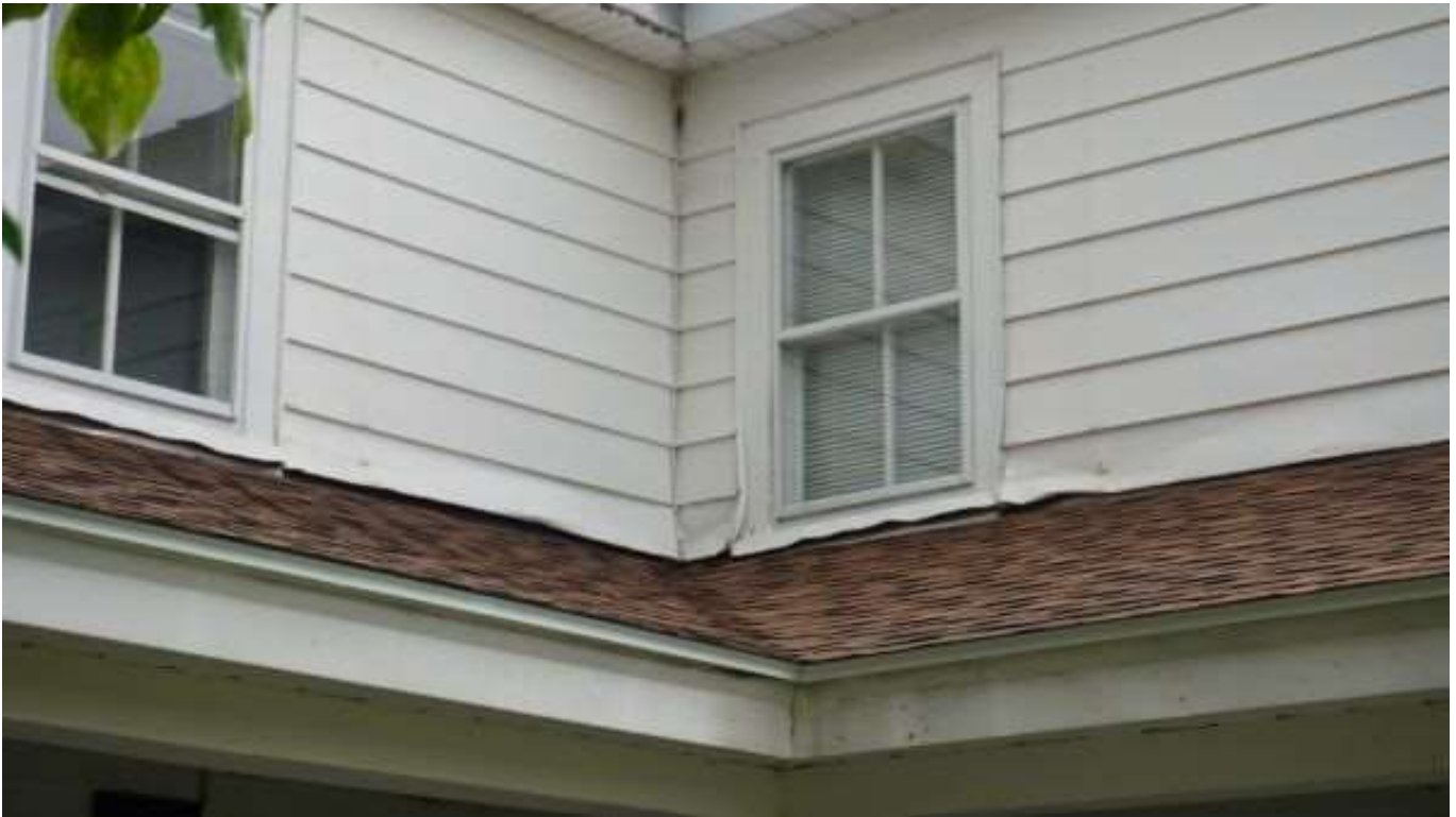
Below: Front porch roof – drip edge present
