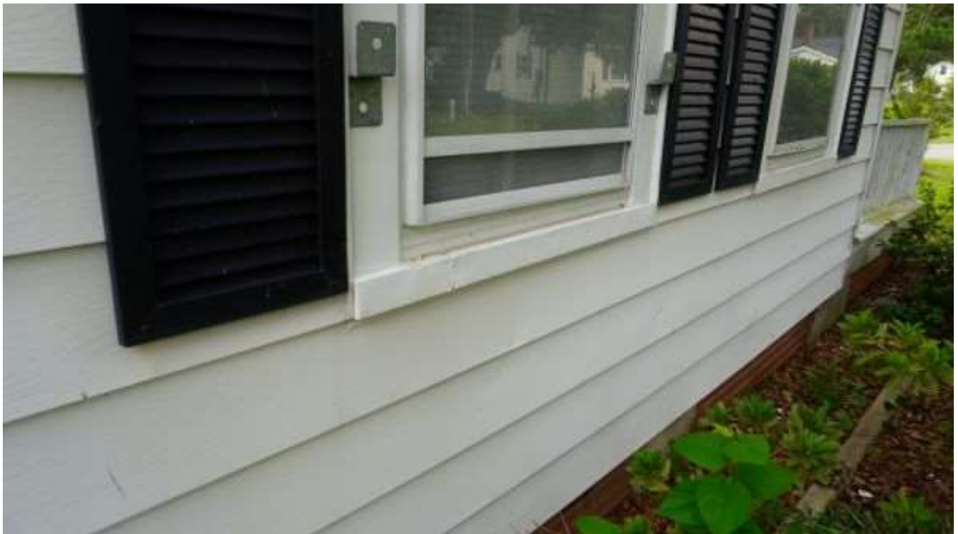
Below: Left elevation – siding scrapes and dents not apparently related to loss
