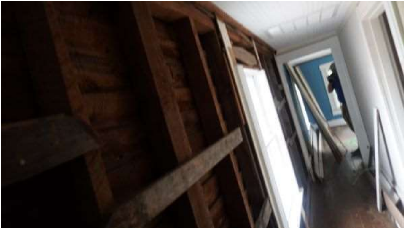
Below: Interior – upstairs hallway – paneling removed – porch roof framing visible
