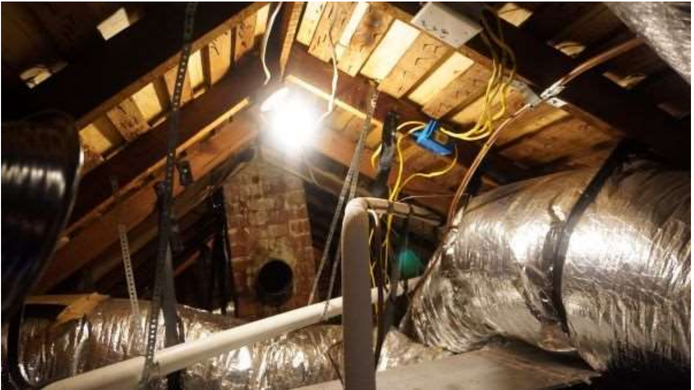
Below: Attic – Roof farming with spaced and solid decking visible
