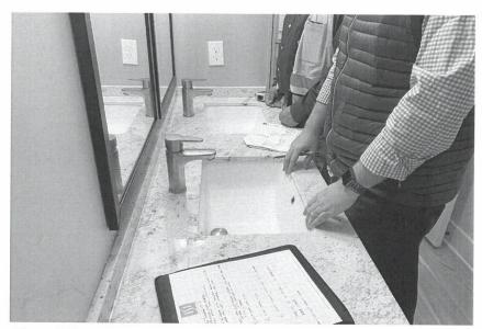
Above: 27" spacing with two grown men showing ample space for use. Below: Required ANSI clear floor space shown at both sinks.
