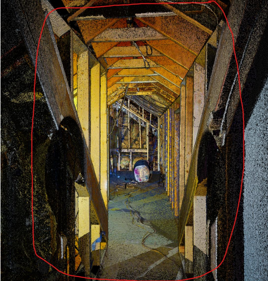
Figure B-3 – Hallway Centerline Headroom (Point-Cloud Interior View)
