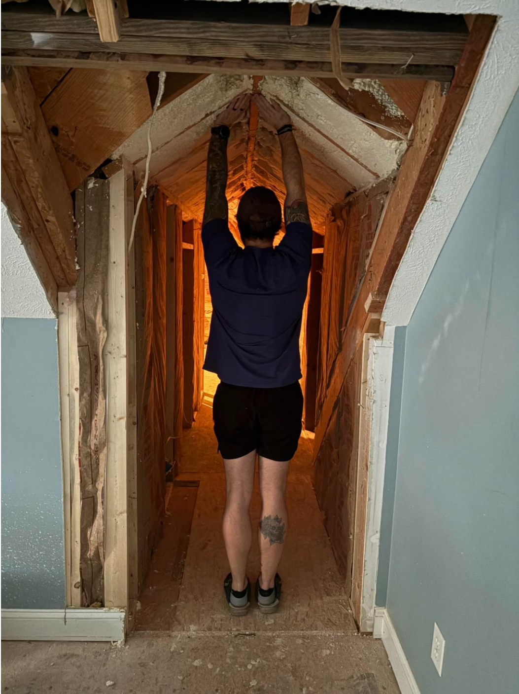
Figure B-6 – Interior Photograph Demonstrating Functional Headroom
