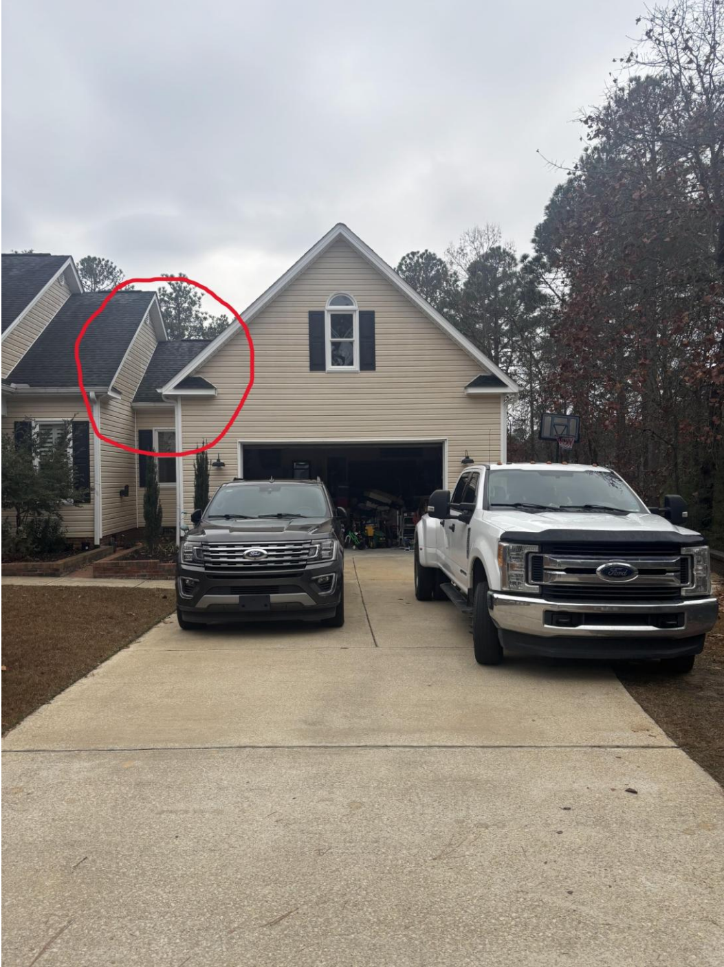
Figure B-5 – Exterior View of Existing Dormers and Roof Planes
