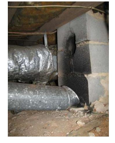
Failing to identify a detached duct;
